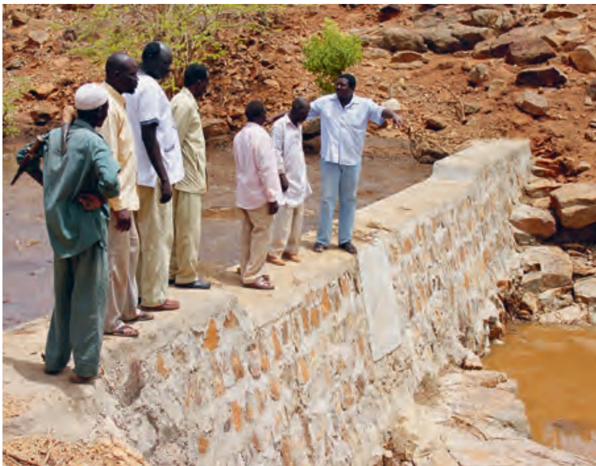
Introducing sand dam technology to Damba village in South Kordofan, Sudan.
