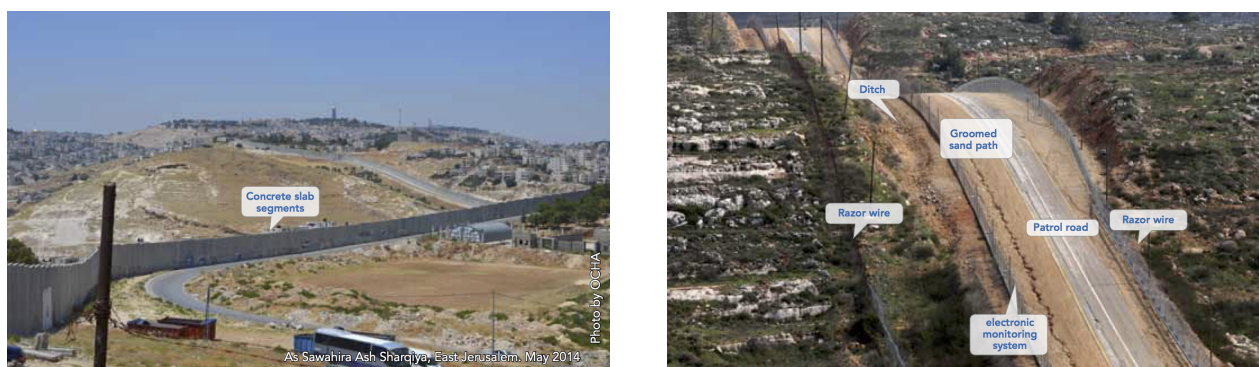
(a) Concrete barrier
